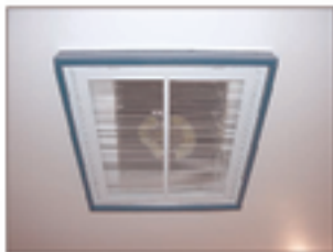
Figure 4.6a — Sheet duct boot, grille closed
